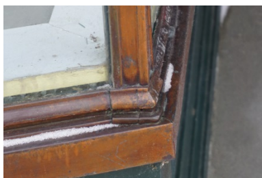
Original storefront detail.
