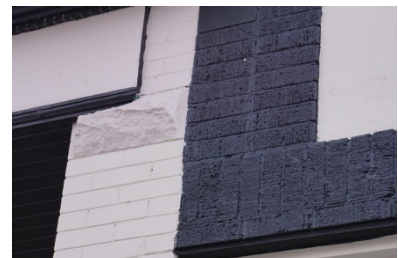
A large percentage of the brick surfaces in the HCD have been painted. Avoid painting masonry or using abrasive cleaning techniques.
