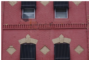
Elaborate brick detailing should be preserved.
