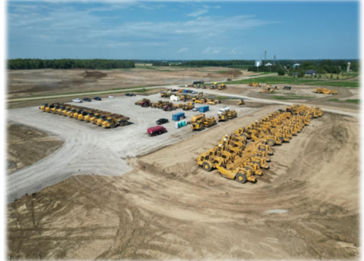
Contractors Equipment - Now Fully Mobilized - July 5, 2023
