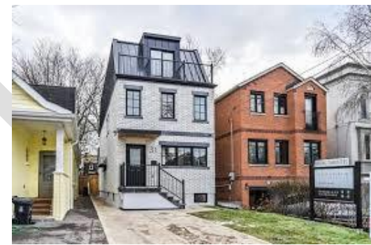
Figure 19 - Neighbourhood streetscape (image credit: OHBA.ca)
