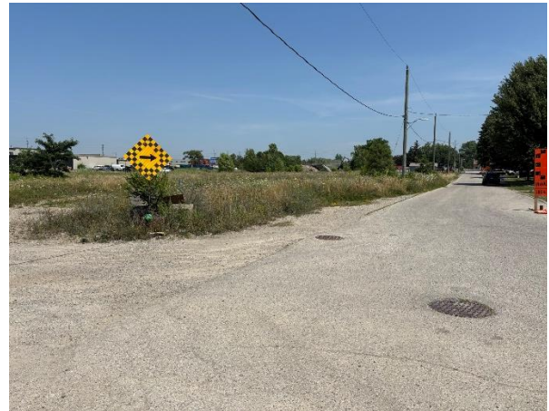
Photograph 2 – Existing Warehouse Street, looking east from the Warehouse Street/Park Avenue intersection.
