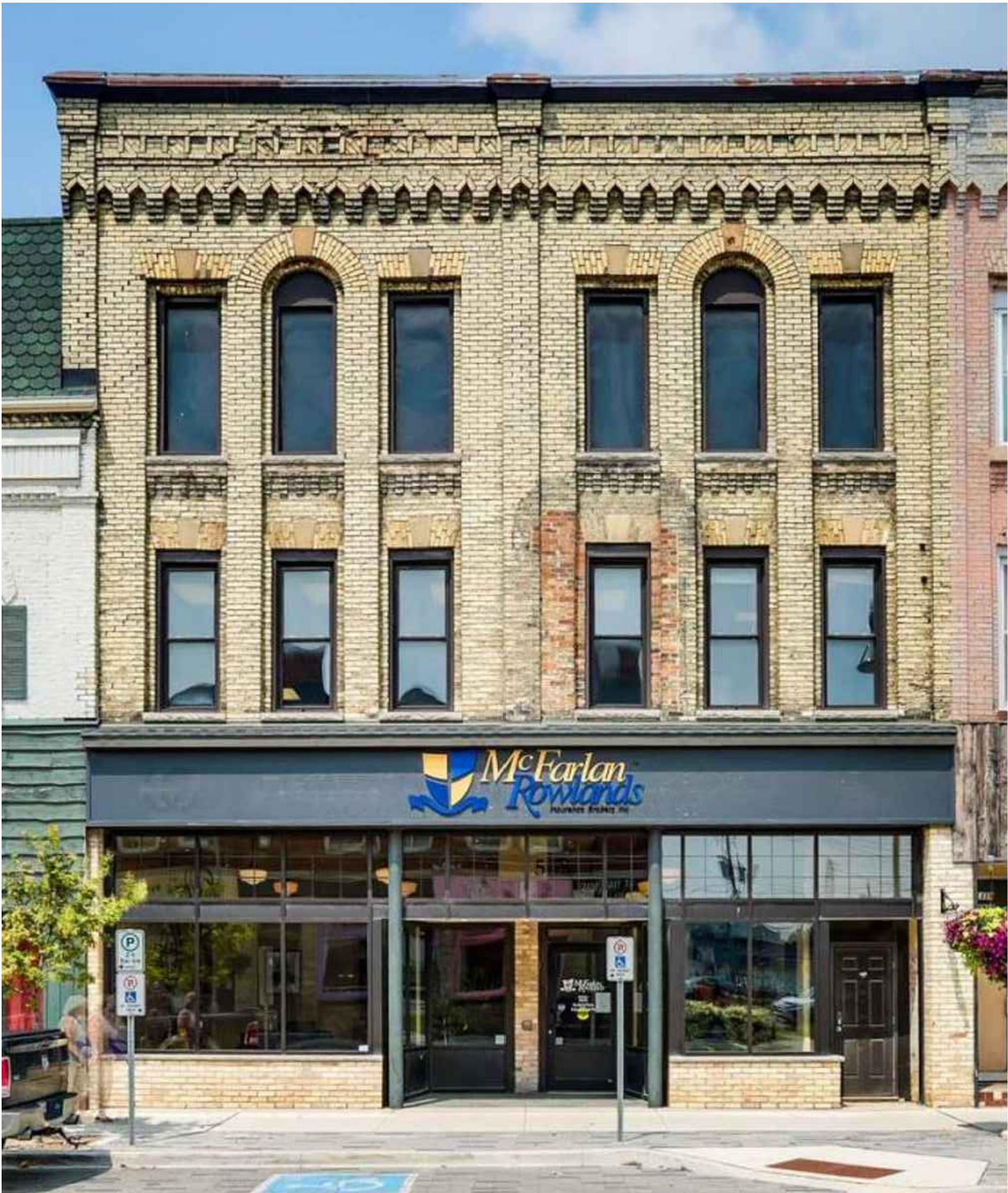
EXISTING BUILDING FACADE
