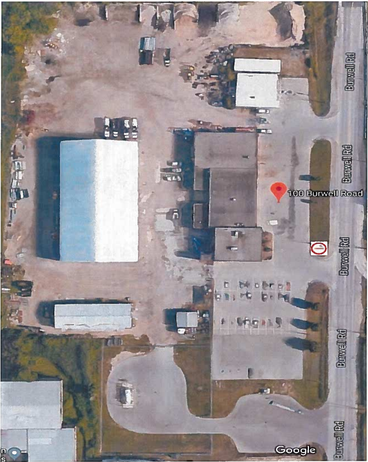
SEWAGE Pollution Control Plant, 40359 Bush Line
