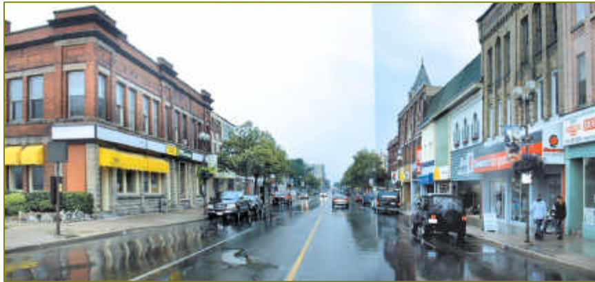
View along Talbot Street at Princess Ave/St. Catherine Street looking west
