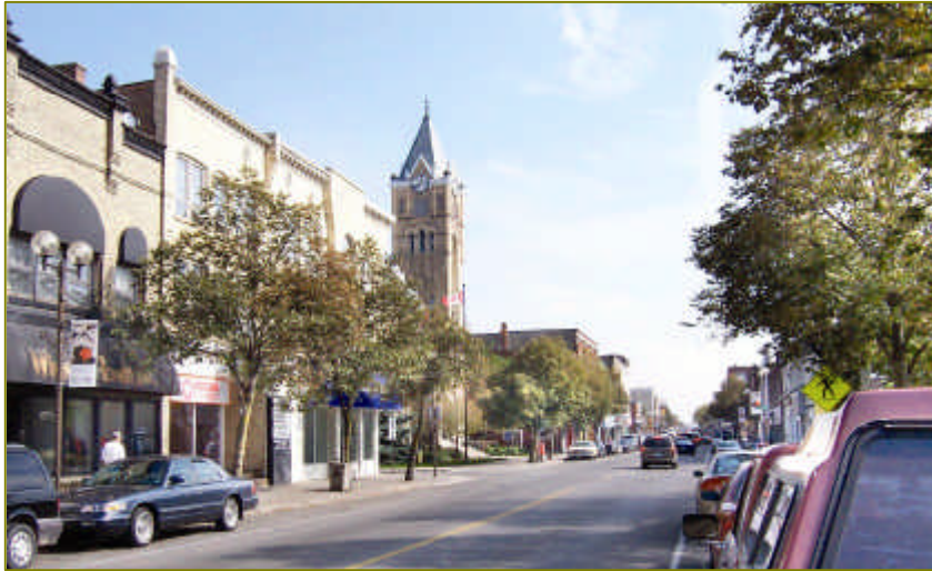
View Along Talbot Central – Potential for a Pedestrian Focused Shopping Retail Area
