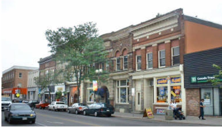
Variety of Treatment at Retail Display Windows and Entrances
