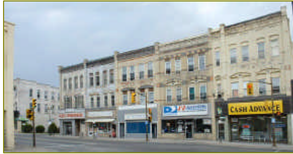
Three Storey Heritage Facades
