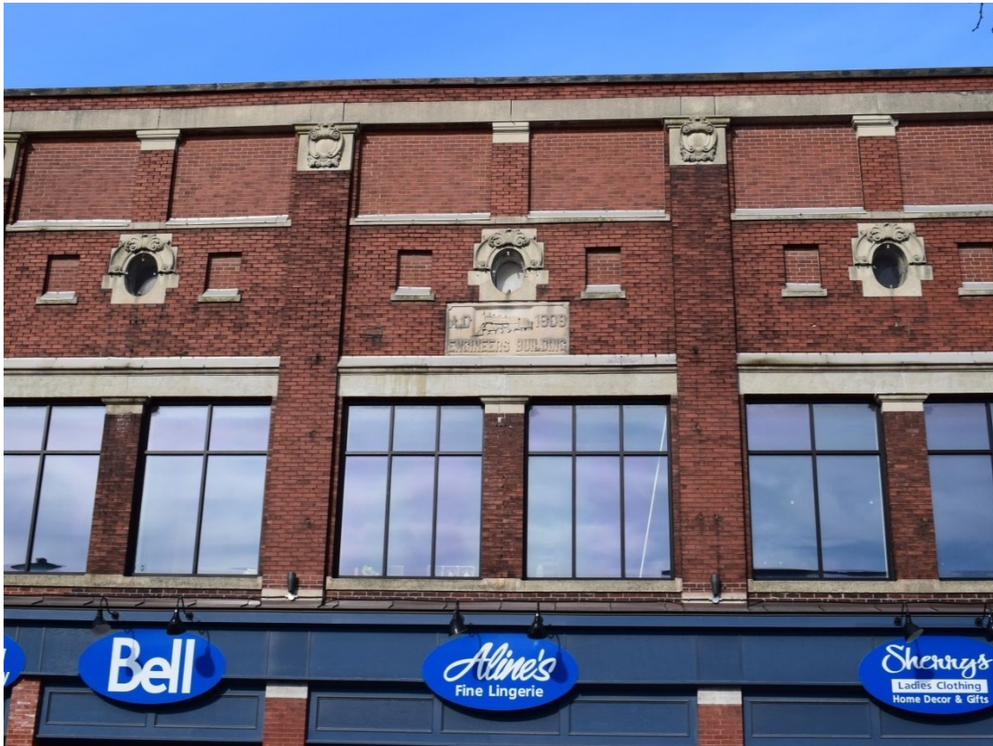
Plate 21: Detail of the Engineer's building.
