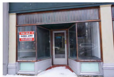
Storefront with original metal framing, wooden panels and glazing.
