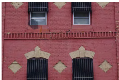
Elaborate brick detailing should be preserved.
