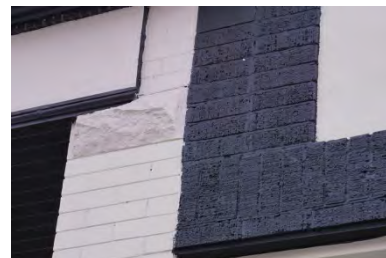
A large percentage of the brick surfaces in the HCD have been painted. Avoid painting masonry or using abrasive cleaning techniques.
