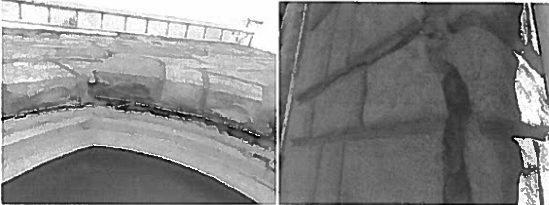
Exterior faux stone pulling away from brick behind (both pics, water infiltration)
