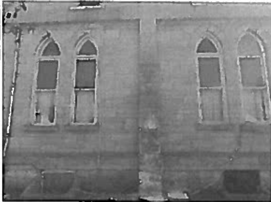
Buttress damaged (faux stone and brick damaged, water infiltration)
