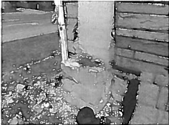
Buttress total collapse
