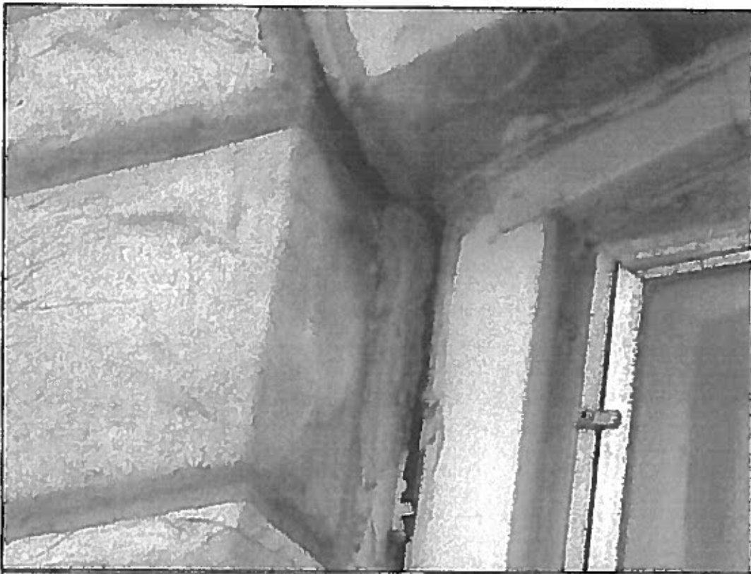
SHOWS EXTERIOR FACADE HAS CRACKED FROM THE SOFFIT TO THE FOUNDATION
