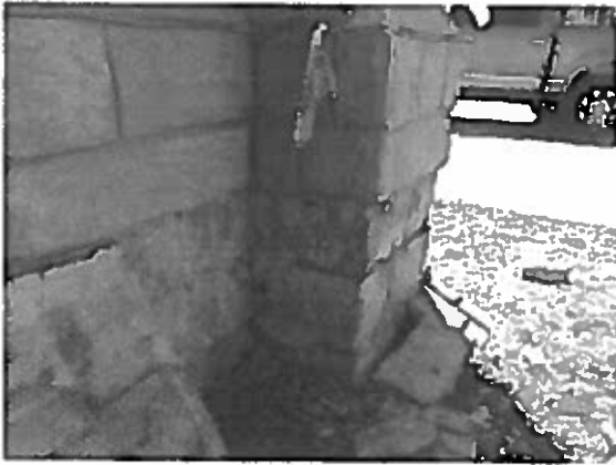
Buttress damaged (faux stone and brick damaged, water infiltration)
