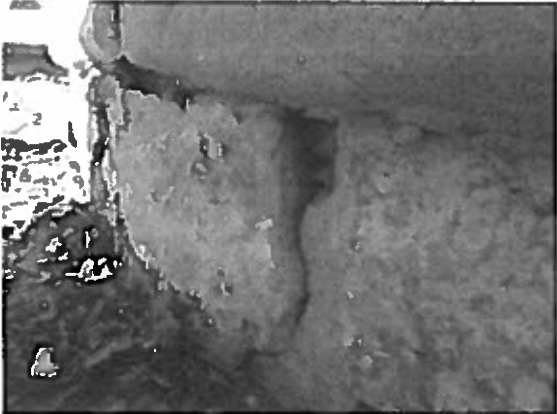
Foundation stone damages (water infiltration)
