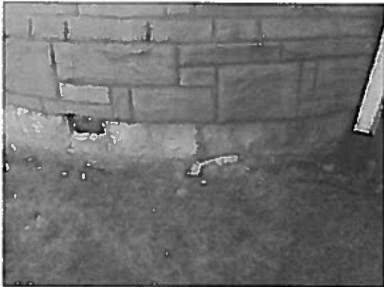
Buttress damaged (faux stone and brick damaged, water infiltration)
