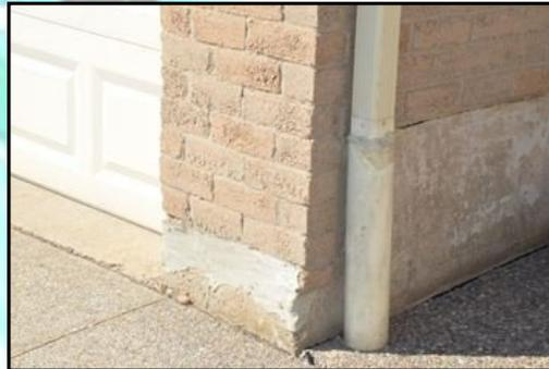
If the downspouts and weeping tiles are connected into the sanitary system they **must** be disconnected at the surface.
