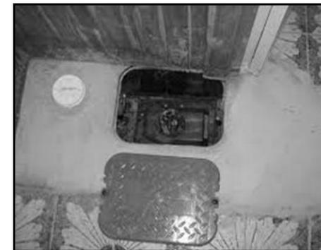
Before opening a sewer BWV put on rubber gloves. Any brushes used to clean the valve must be bleached or only used for this one purpose and stored in a safe place between uses. After completion, discard gloves and wash hands thoroughly as well as clothes.
