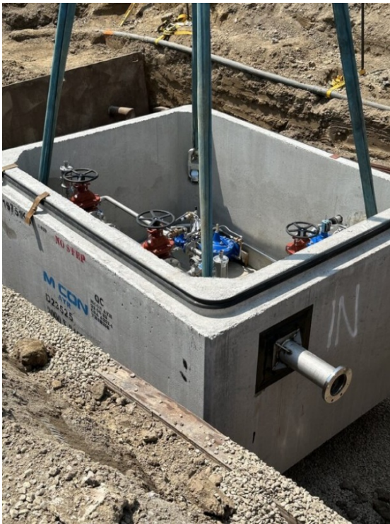
Figure 4: Installation of a new pressure reducing valve chamber.
