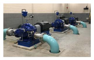
The three high lift pumps provide redundant pumping capacity into the STASWSS. The St. Thomas pumps are equipped with variable frequency drives (VFD) with each pump having a rated capacity of 263 L/s. With the current VFDs being utilized as soft and stop variable frequency drives.
