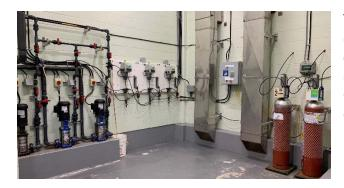
The AASWSS and STASWSS both utilize a gas chlorination system for secondary disinfection. The system consists of two scaled 68 kg gas chlorine cylinders and three chlorinators equipped with booster pumps and a dosing capacity of 1-60kg/h.
