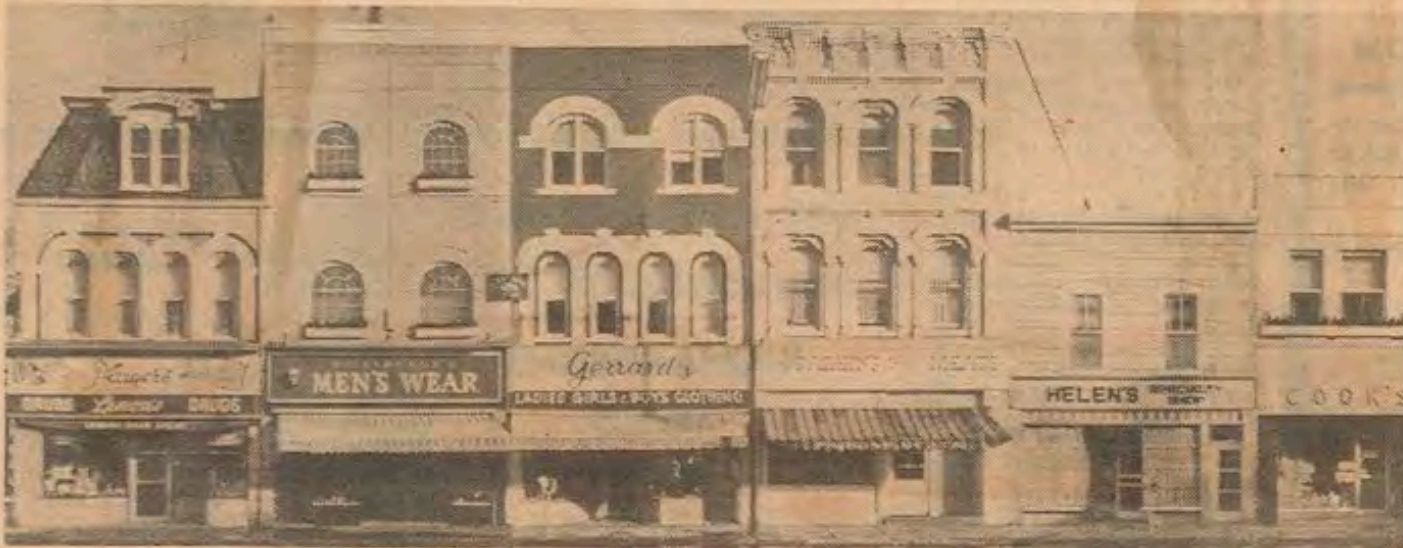
AFTER — Less than four months after work was started this nearly completed view stood out to s
