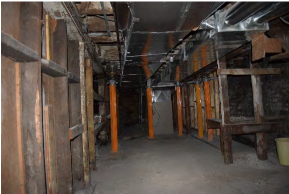
Plate 36: Basement of 248 Talbot Street, looking north
