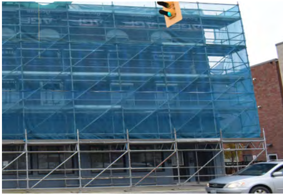
Plate 16: Front façade of 244 Talbot Street, looking south
