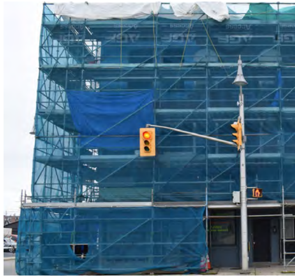
Plate 21: Front façade of 248 Talbot Street, looking south
