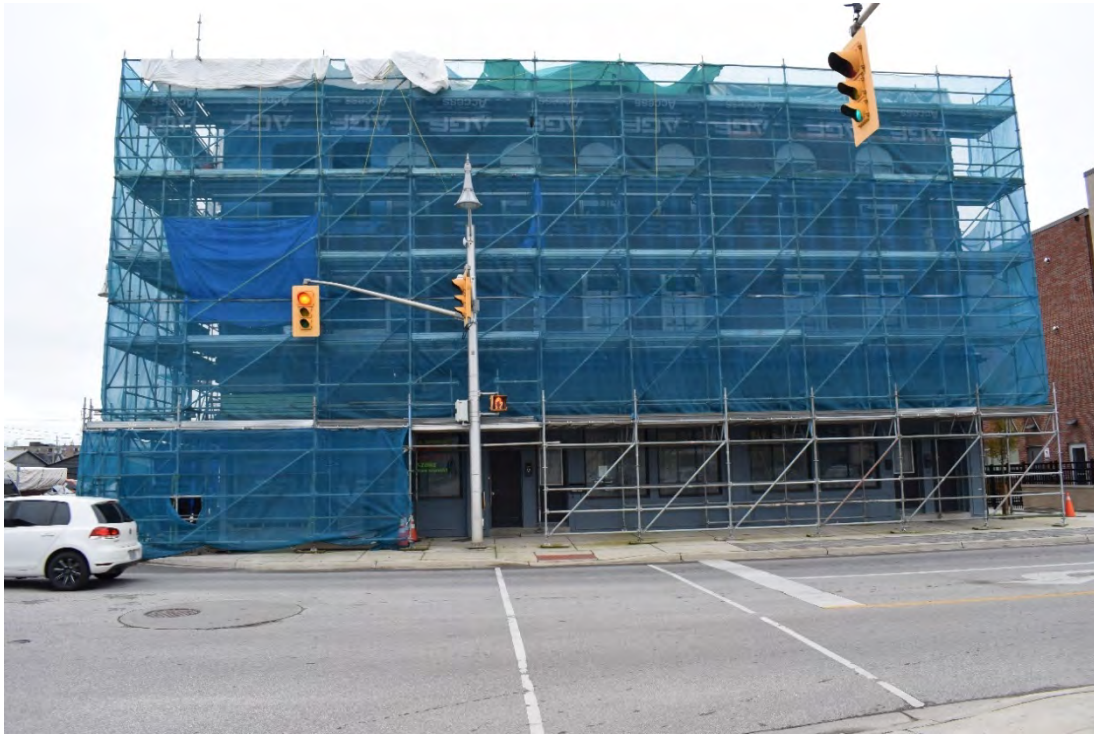
Plate 15: Looking south at front façades, from east to west, 248, 246, 244 Talbot Street
