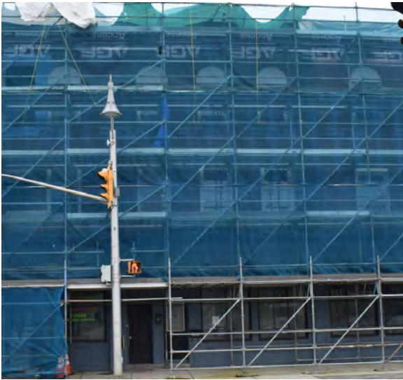
Plate 20: Front façade of 246 Talbot Street, looking south
