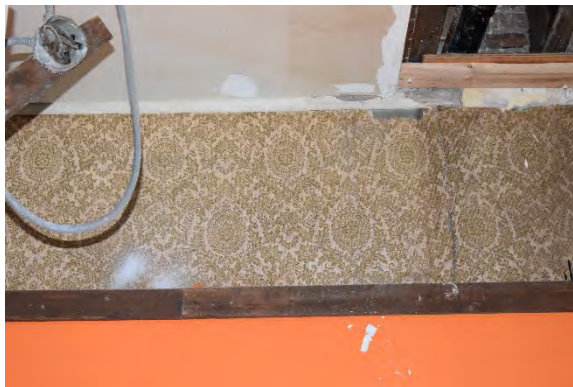
Plate 35: Wallpaper above drop ceiling, looking west
