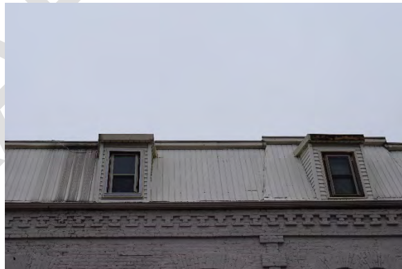
Plate 23: Details of mansard roof, dormers, and corbel on 248 Talbot Street, looking west
