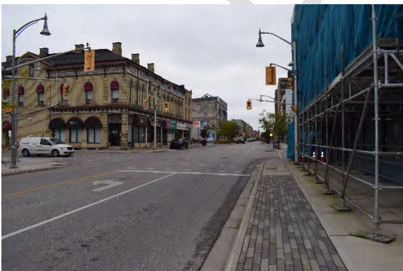
Plate 10: Looking east at intersection with 244, 246, and 248 Talbot Street at right
