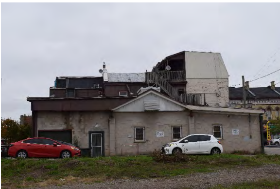
Plate 26: North addition, 244 and 246 Talbot Street
