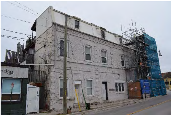
Plate 22: East elevation, 248 Talbot Street, looking northwest
