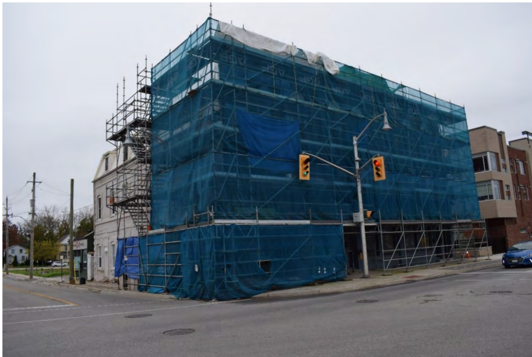
Plate 14: Scaffolding partially obscuring views, looking southwest
