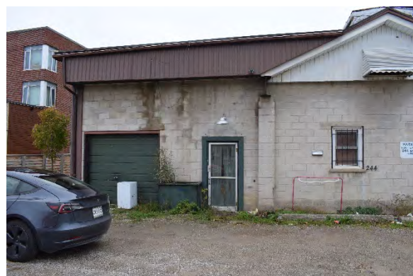
Plate 29: Looking north at garage, door, and window
