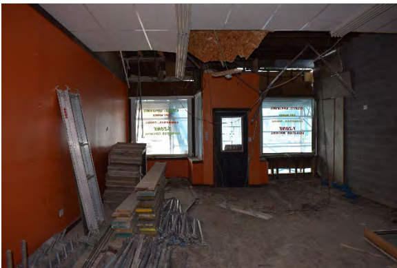
Plate 34: First storey of 248 Talbot Street, looking north
