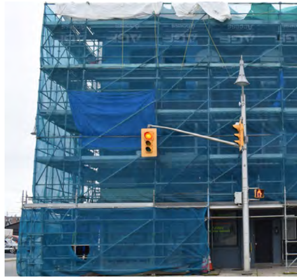
Plate 21: Front façade of 248 Talbot Street, looking south
