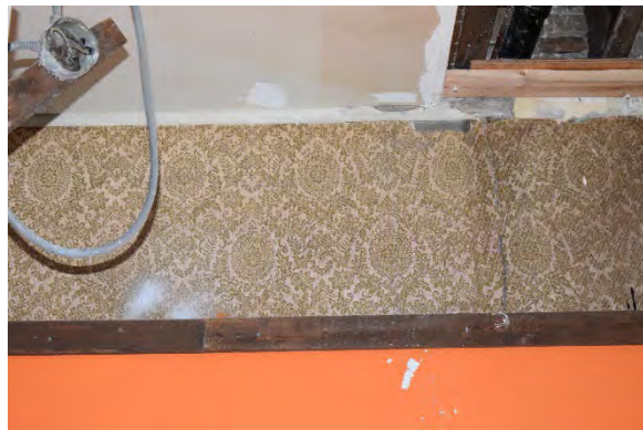
Plate 35: Wallpaper above drop ceiling, looking west
