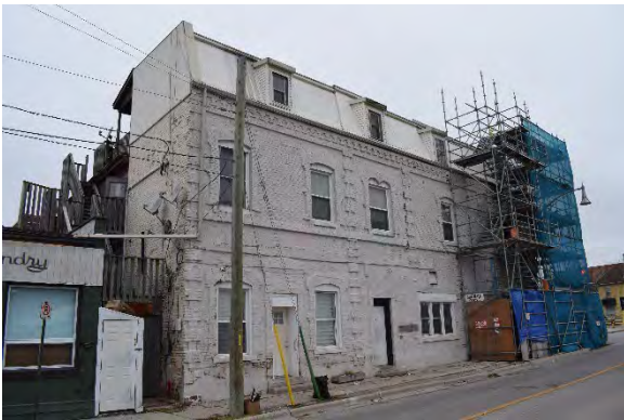
Plate 22: East elevation, 248 Talbot Street, looking northwest
