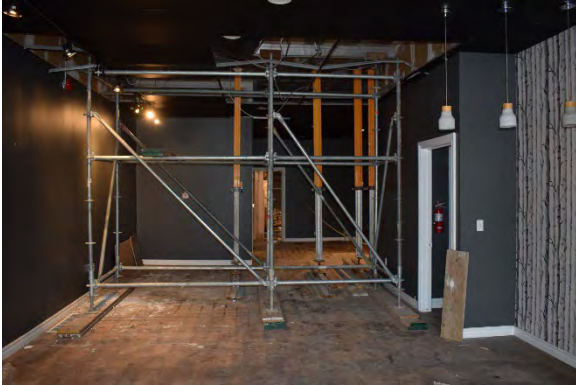
Plate 30: First storey of 244 Talbot Street, looking south
