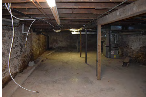
Plate 31: Basement of 244 Talbot Street, looking north
