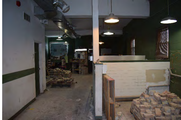
Plate 37: Interior of former laundromat, looking east
