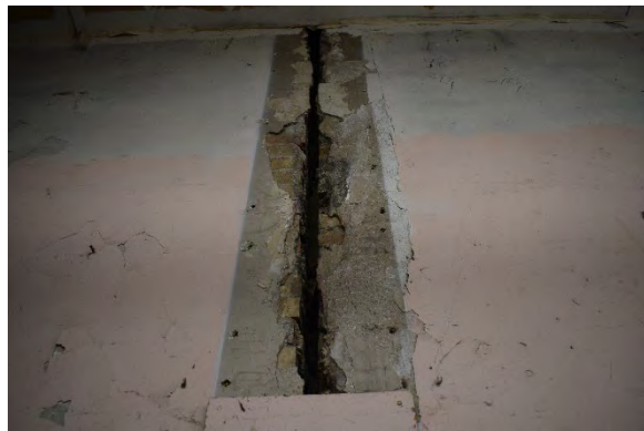
Plate 41: Wall gap, looking east
