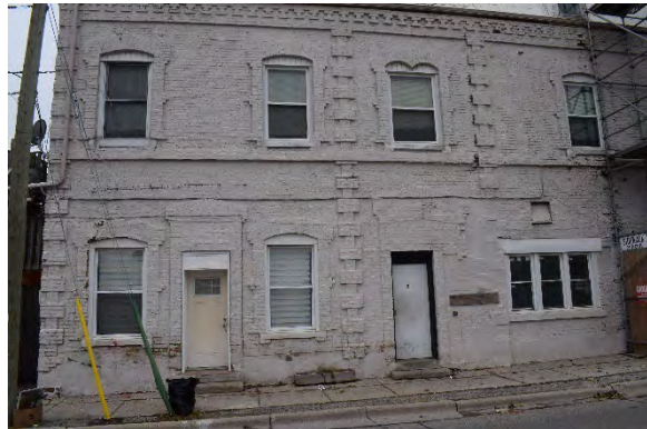
Plate 25: Details of first storey, 248 Talbot Street looking west
