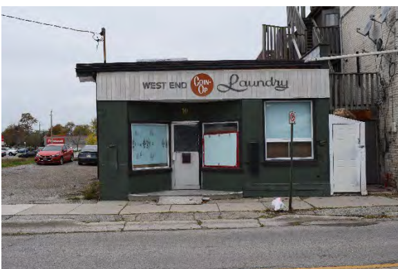
Plate 28: Storefront details, looking west
