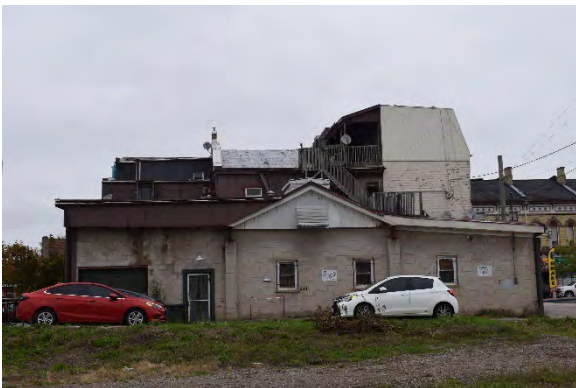
Plate 26: North addition, 244 and 246 Talbot Street
