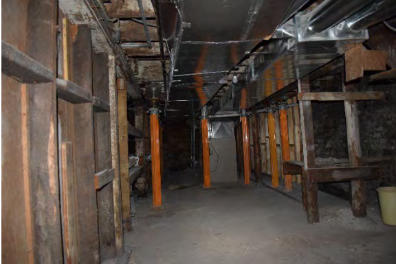
Plate 36: Basement of 248 Talbot Street, looking north
