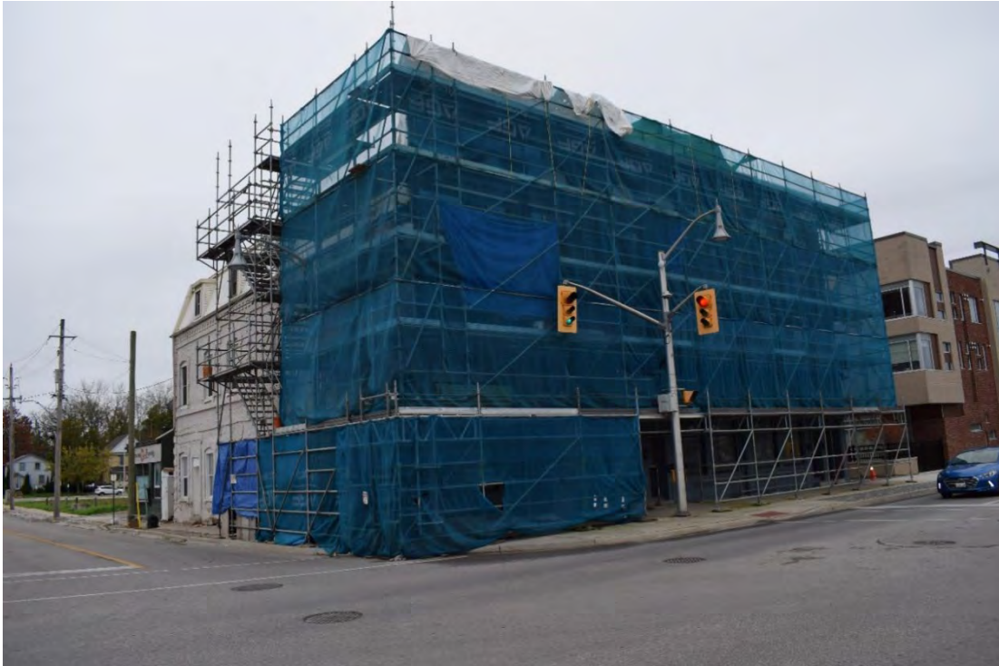
Plate 14: Scaffolding partially obscuring views, looking southwest
