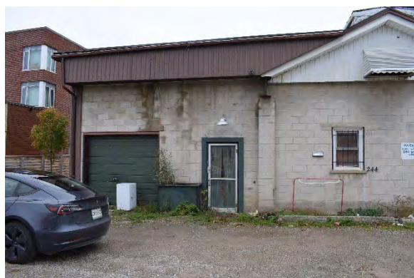
Plate 29: Looking north at garage, door, and window
