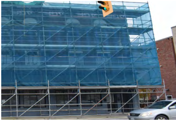
Plate 16: Front façade of 244 Talbot Street, looking south
