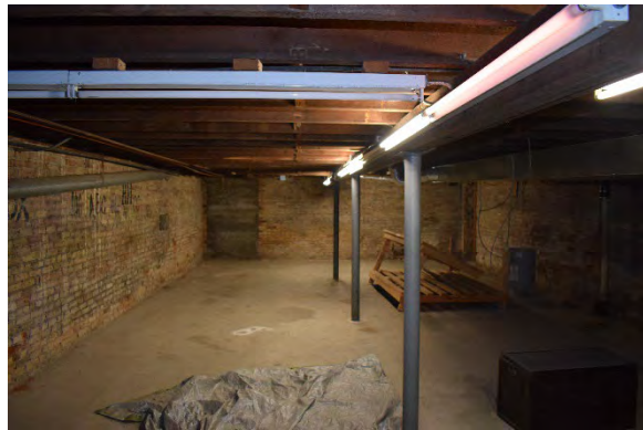
Plate 33: Basement of 246 Talbot Street, looking north
