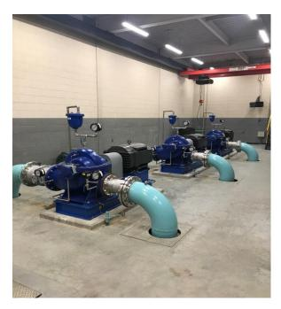
The St. Thomas pump station is comprised of three high-lift pumps that deliver water through a transmission main that services the St. Thomas Area Secondary Water Supply System. A gas re-chlorination system provides re- chlorination for water being directed to the St. Thomas Area Secondary Water Supply System.
