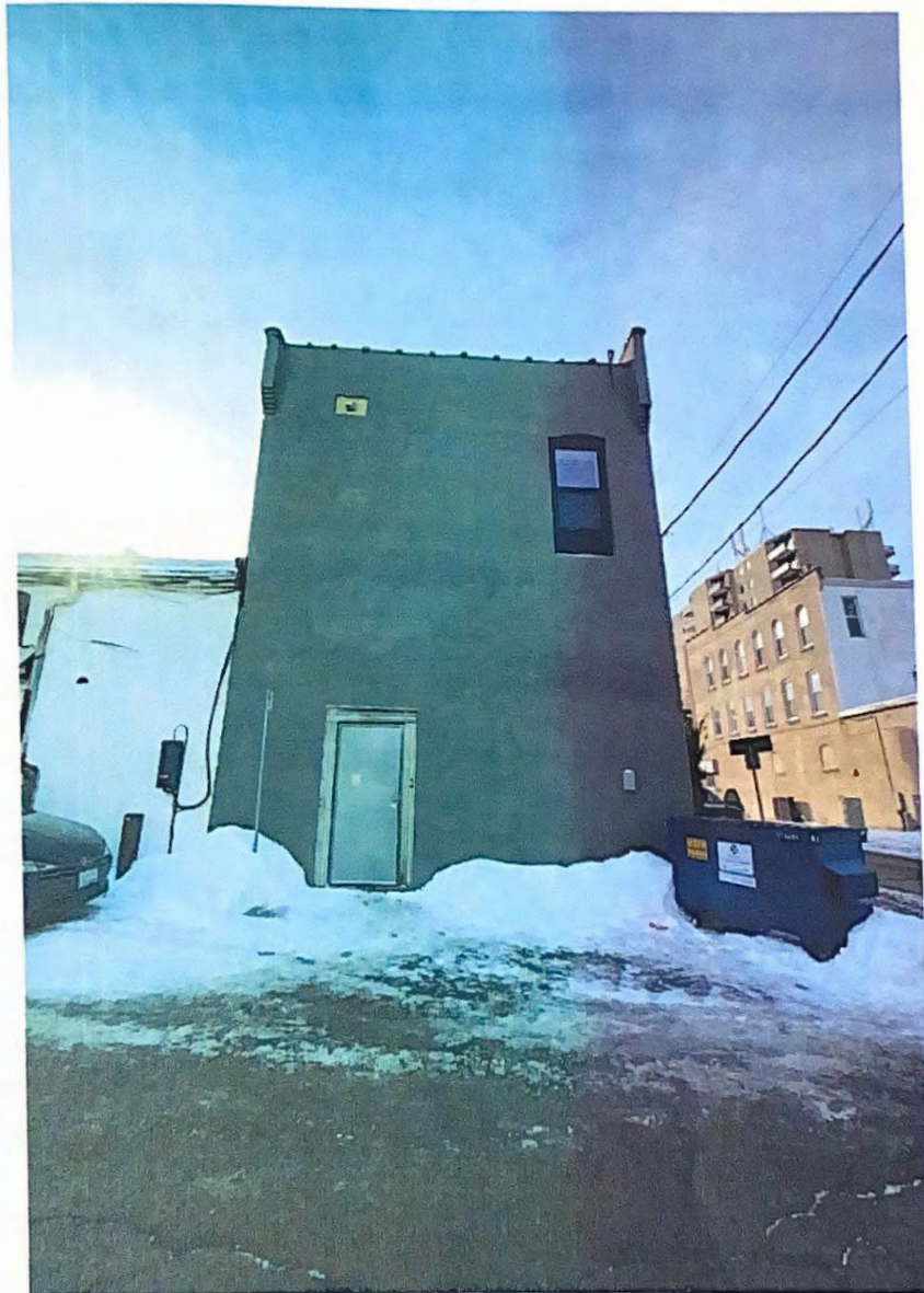
Figure 1 - Rear Wall of 341 Talbot Street
