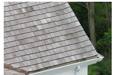
7.5 MONITOR EAVESTROUGHS &amp; DOWNPIPES
