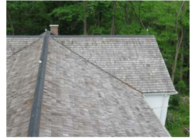
7.1 CEDAR SHINGLE ROOF
