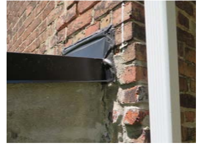
6.3 REPOINT BRICK AT REGLET CONNECTIONS
