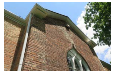
6.2 REPOINTING AT SOUTH WALL
