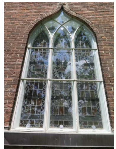
5.2 NEW LEXAN PANELS AND VENTS INSTALLED ON SOUTH WINDOW
