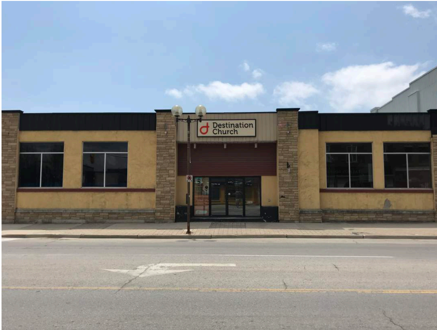
North Elevation (photo) of Destination Church Facade - Photo Taken June 29, 2021
