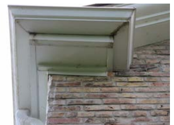
7.4 MONITOR EAVESTROUGHS &amp; DOWNSPOUTS
