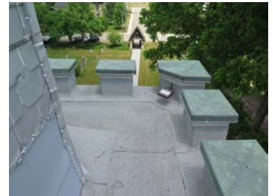
8.3 COPPER CAPS IN GOOD REPAIR
