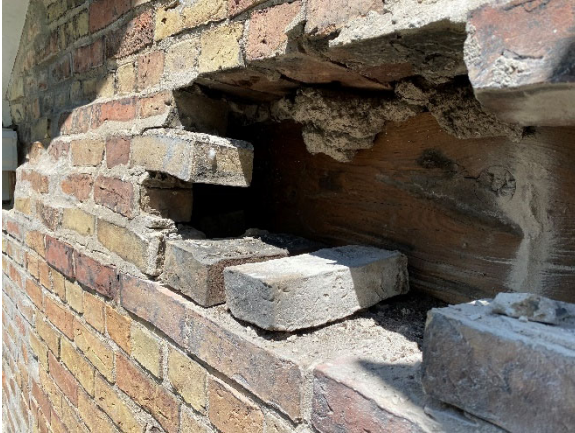
Masonry Inspection Opening Header course
