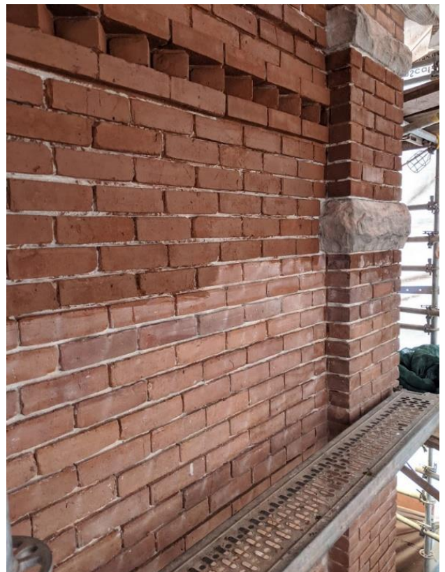
Figure 2 Red Wash applied to historic brick in Toronto, Ontario
