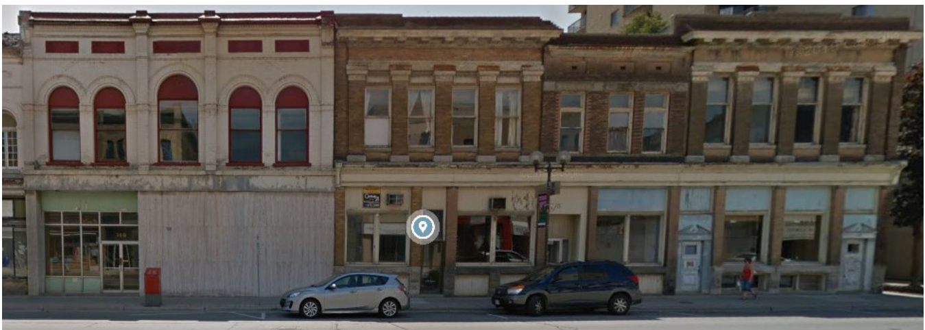
Image 3: North Elevation of Site: 344-360 Talbot Street. Streetview: Google Maps, 2016.
