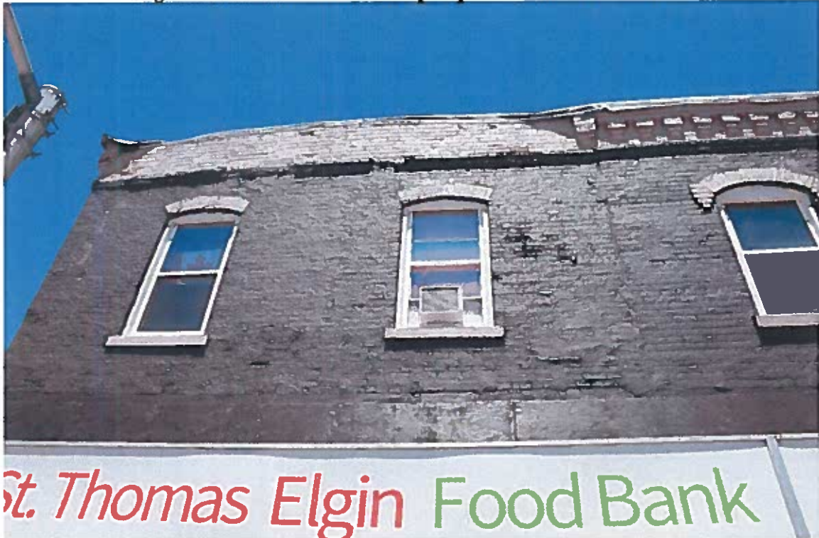
Figure 4. The West section of the parapet wall on South elevation
