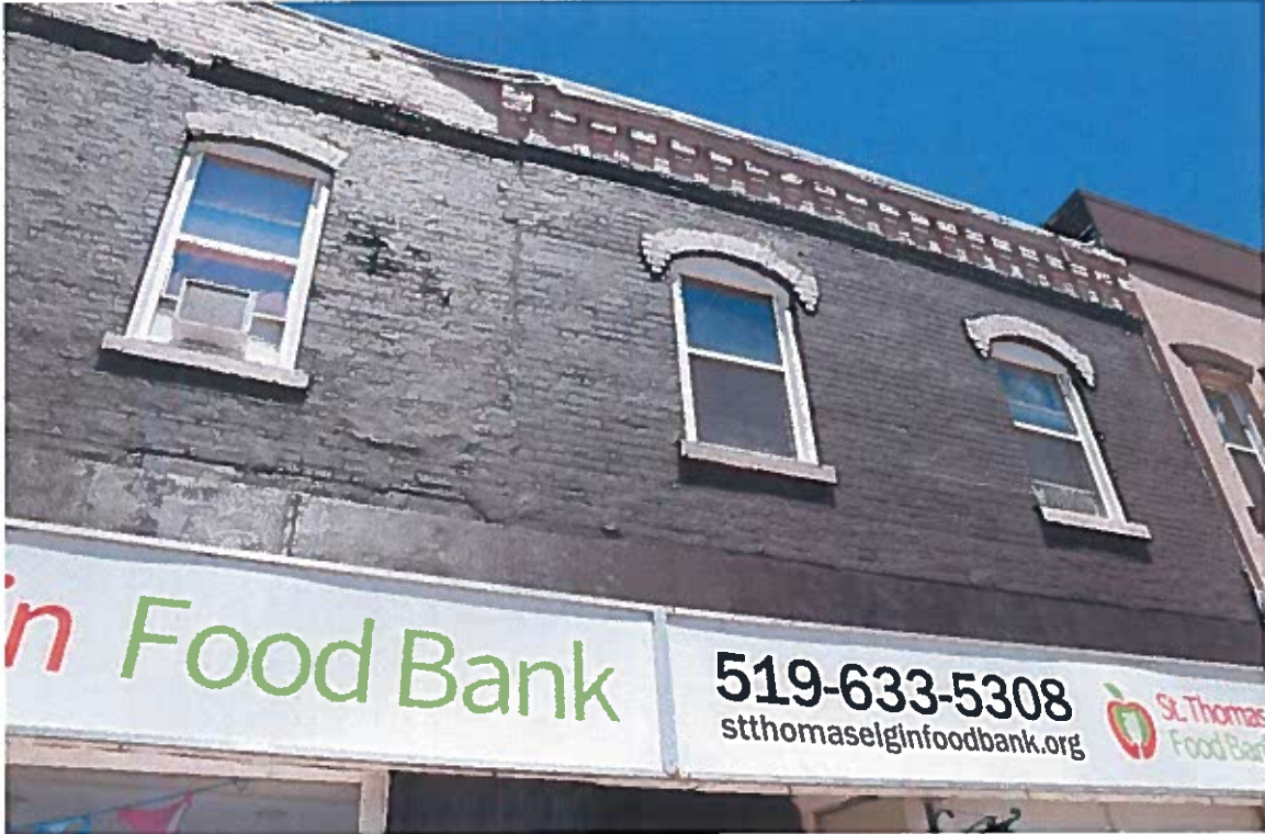
Figure 3. The East section of the parapet wall on South elevation
