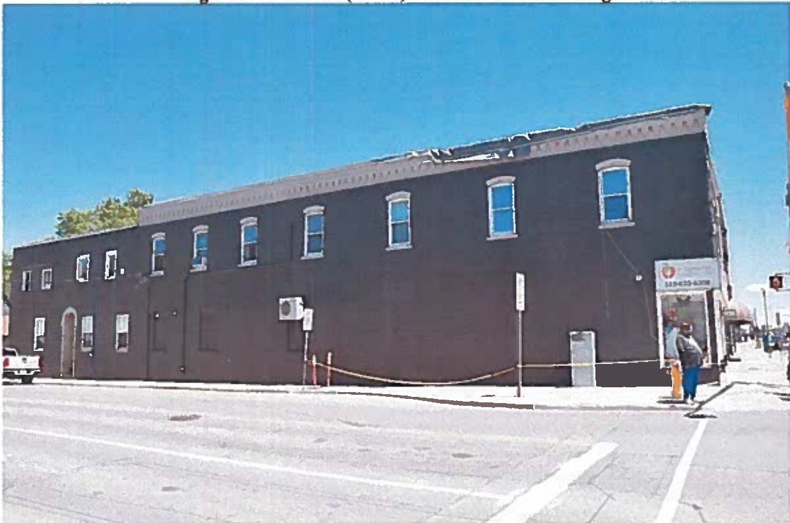
Figure 2. The West elevation of the building
