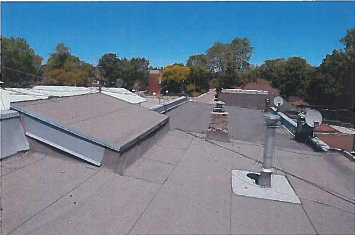
Figure 6. The North / undamaged section of the roof
