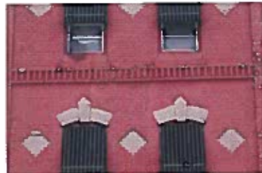
Elaborate brick detailing should be preserved.
