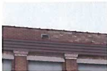
Metal flashing on parapet.
