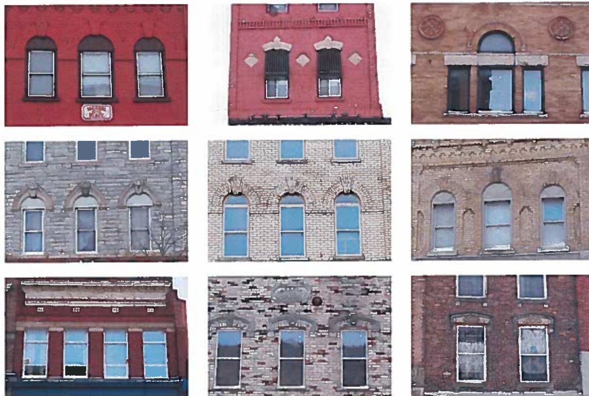
Plate 12: Examples of window types and shapes in the HCD. Rectangular, round arch and segmental arch are most common.
