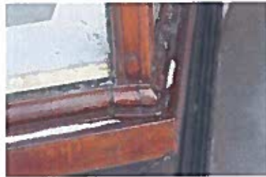
Original storefront detail.
