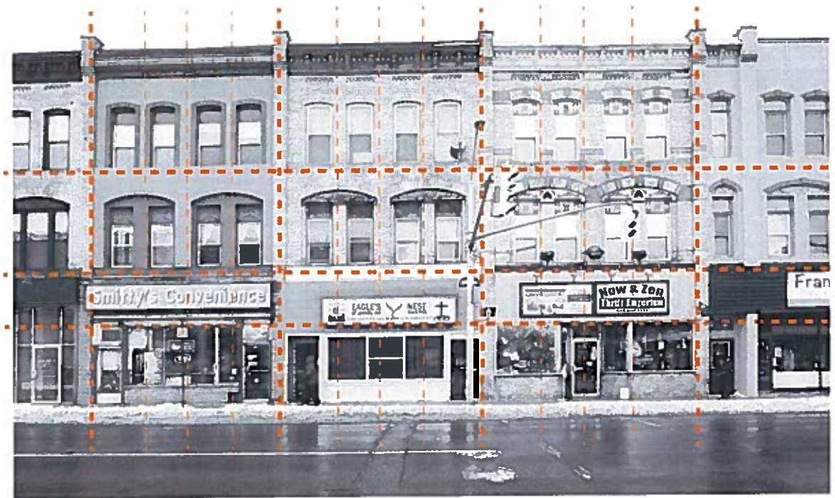
Plate 5: Maintain the rhythm of windows and doors in the façade that make up the traditional commercial/mixed-use façade pattern in the HCD
