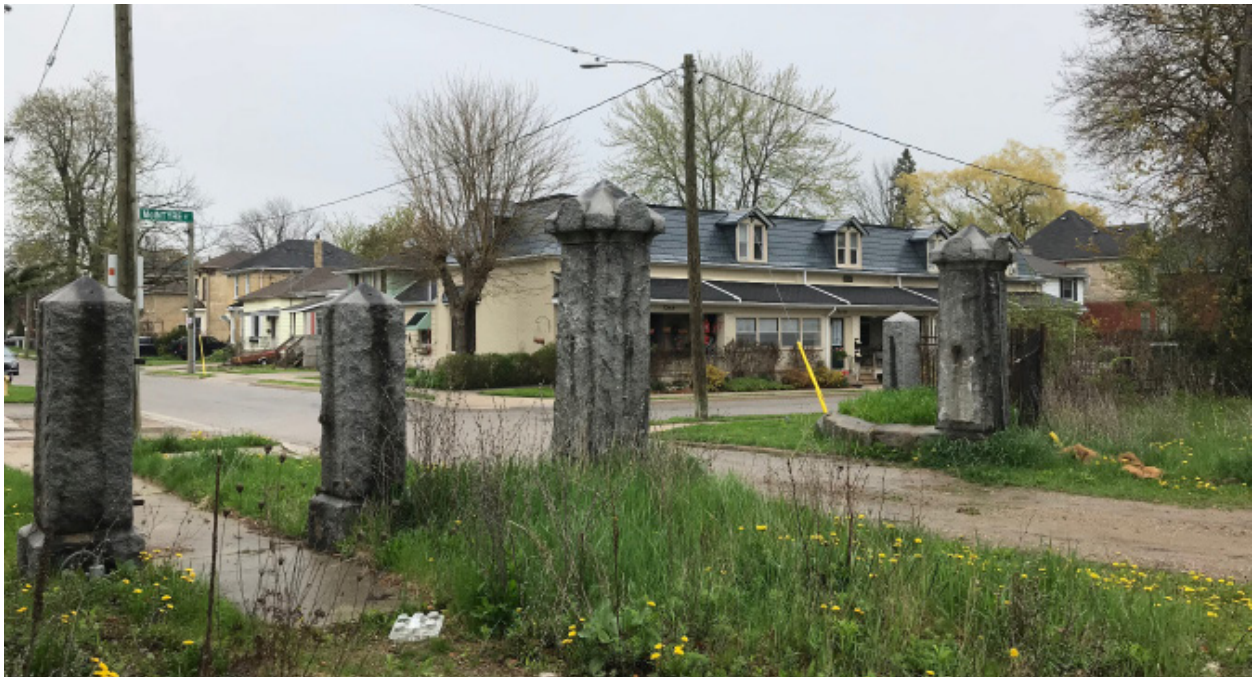
Existing condition of the stone pillars (ERA, 2018).
