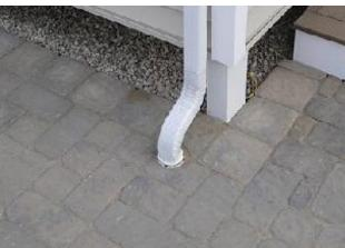
If the downspouts are connected into the sanitary sewage system they **must** be disconnected at the surface. If the downspouts go into the ground you will need to disconnect them and reroute them to allow the water to properly drain from your roof **ONTO** the ground, not **INTO** the ground. A downspout can be disconnected as outlined below.
